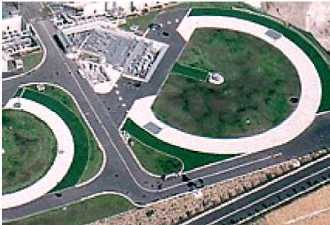
Bird's-eye view of underground storage tanks
