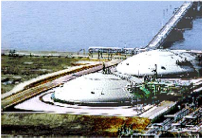
Bird's-eye view of in-ground storage tanks
