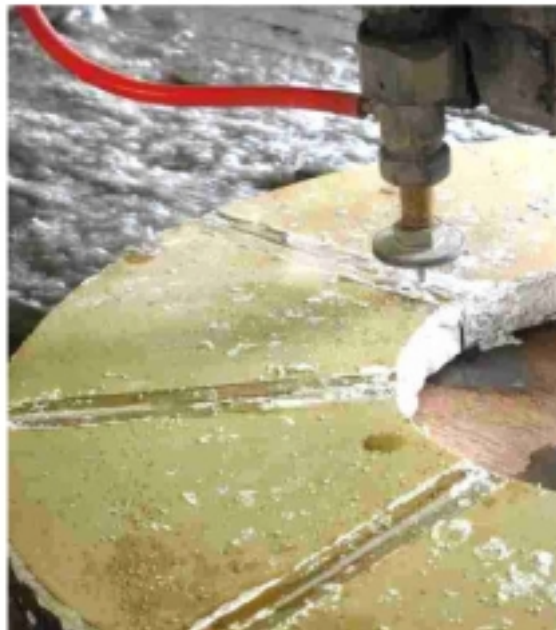
core cutting with water-jet
